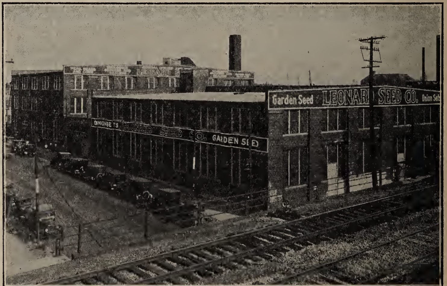
Office and main Chicago Warehouse, 333 to 355 W. 35th St.
